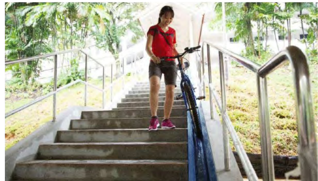
Figure 3.32 Sample Bicycle Wheeling Ramp to be provided adjacent to footpath (Source: www.lta.gov.sg)
