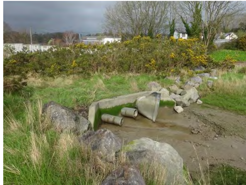
Figure 6.3 – Existing Outfall east of Glounthaune Station at Johnstown Park
