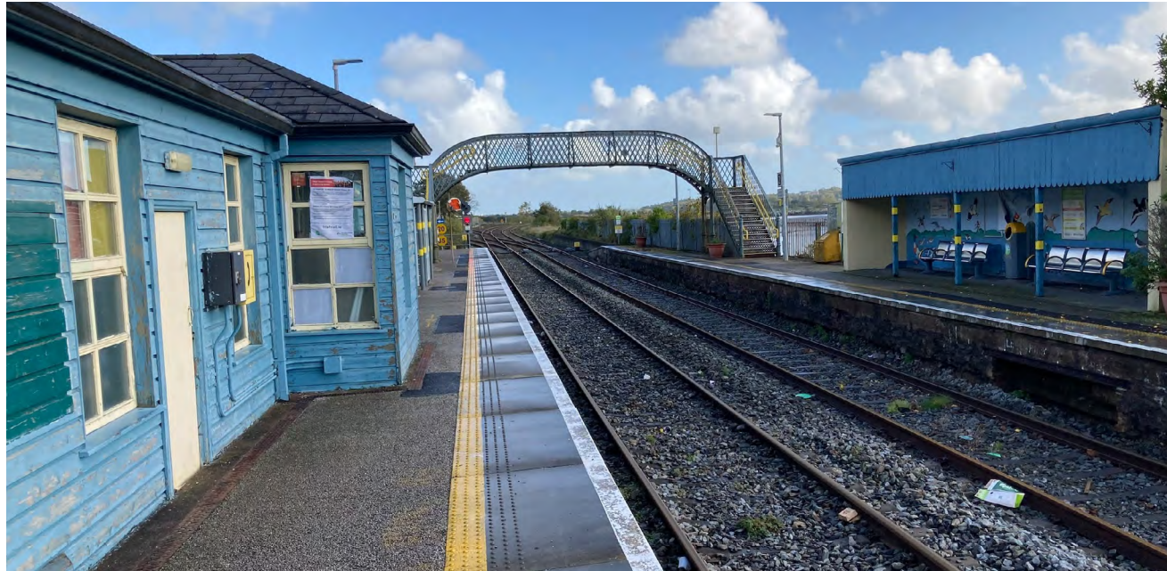
Figure 2.12 Glounthaune Train Station Platform – Looking east towards Cobh, Carrigtwohill and Midleton.
