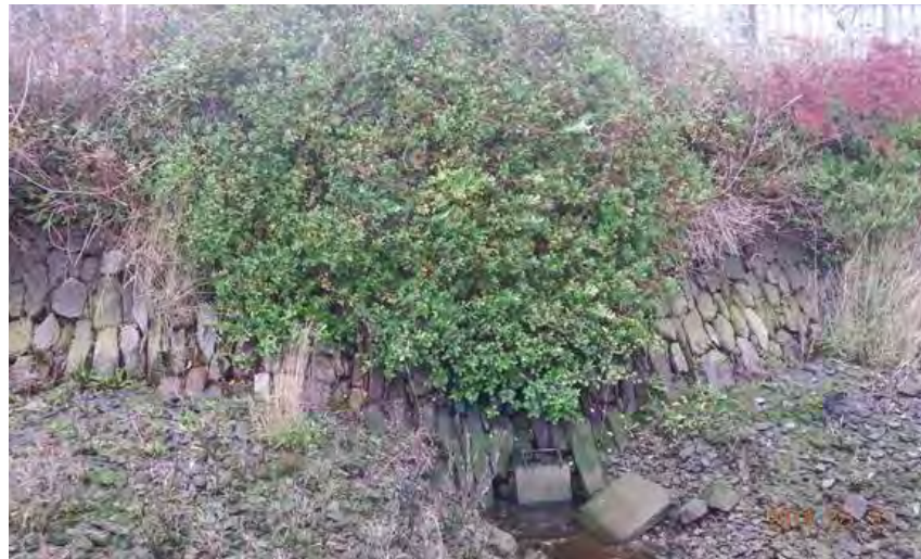
Figure 6.1 – Existing Outfall at Glounthaune Train Station
