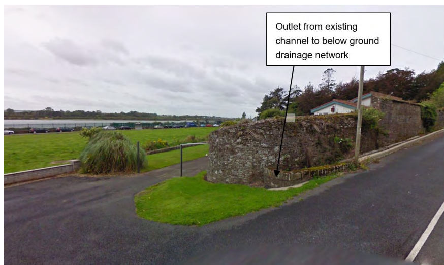
Figure 6.2 – Existing Channel on the Terrace
